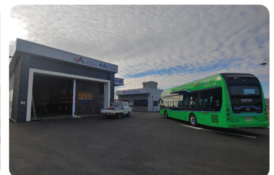
Seosan Fueling Station
