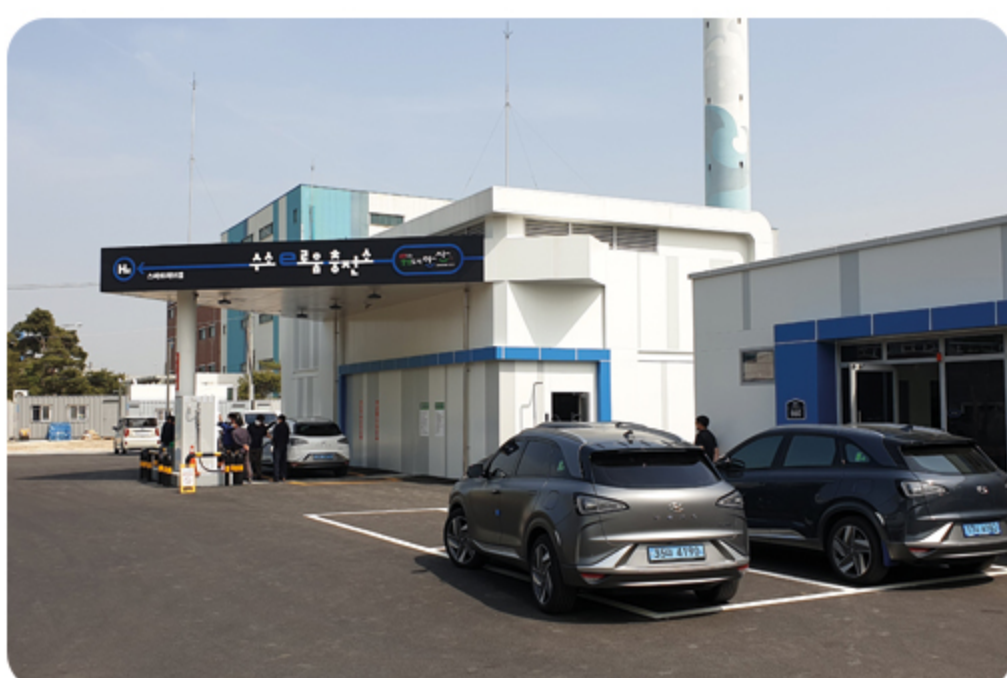
Ansan Fueling Station
